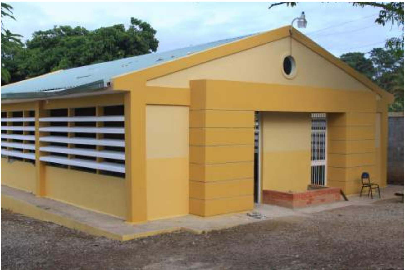
CE La Zanja 08-02 Santiago
